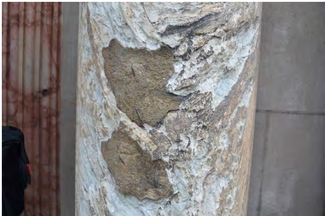
One particularly discolored patch that could be replaced.
