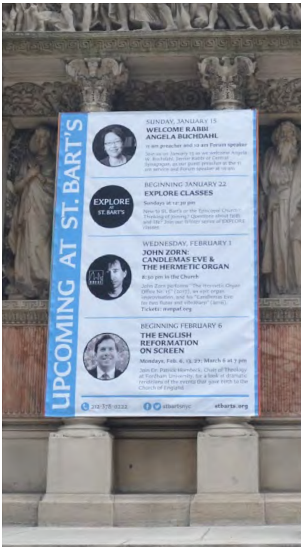
Sign attached to Cipollino columns that should be removed to prevent the wire attachment from abrading the columns any further.
