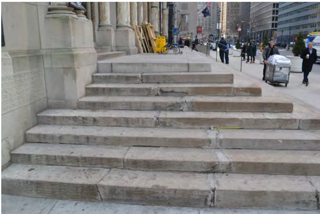
Substantial crack in northwest corner of stairs leading to the portal.
