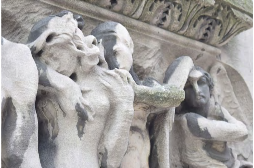
Heavy soiling and jarring contrast between light and dark make the sculpture more difficult to read from ground level.
