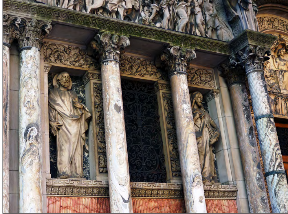
■ Left: Columbia University Graduate Students and Faculty, in collaboration with the Conservancy, examine the Triple Portal conditions. Right: Triple Portal detail highlighting deterioration of the Cipollino marble columns.
