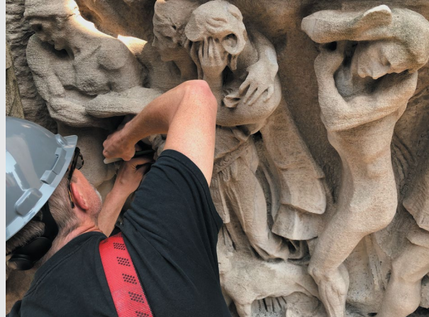
Hands-on Conservation Evaluation from Aerial Lift.
