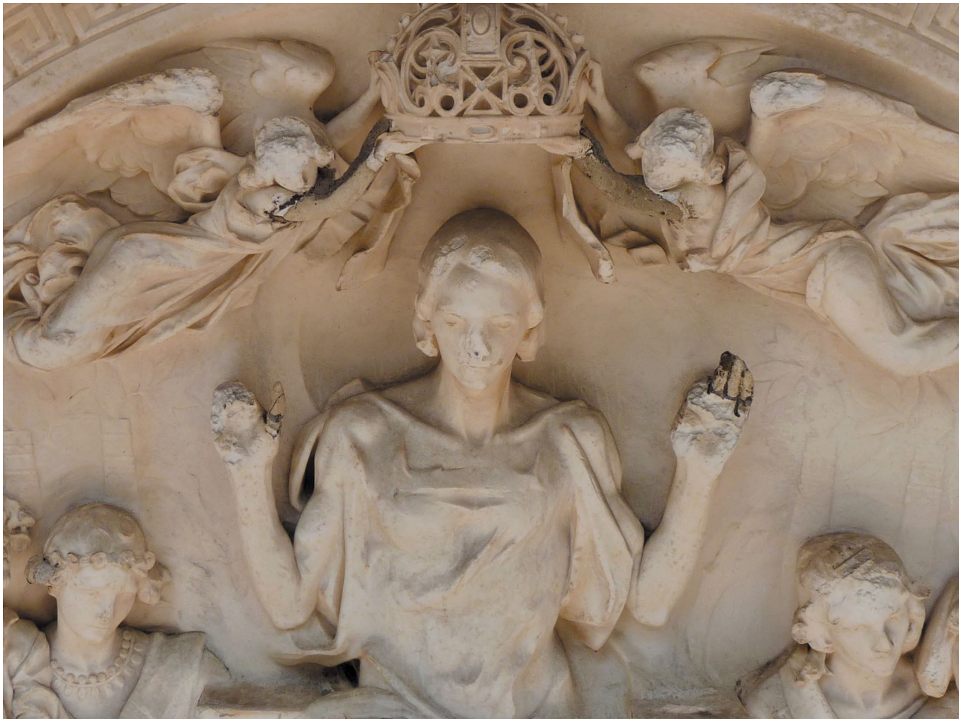
Central Tympanum with Significant Loss of Critical Sculptural Features.
