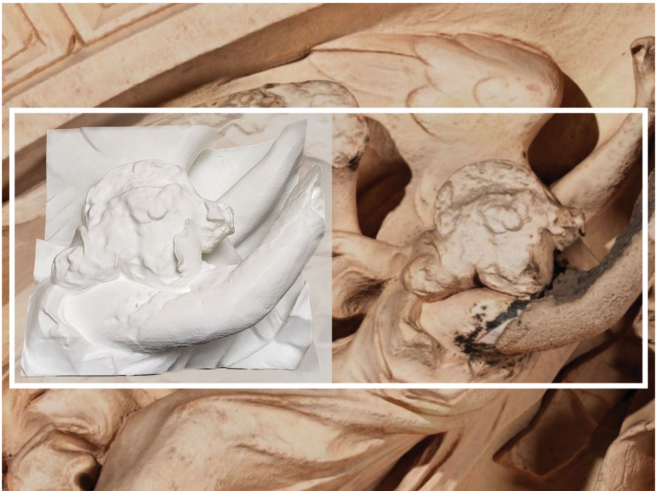
Actual Scale 3D Printed Model (at Left) that Can Support the Restoration Process.
