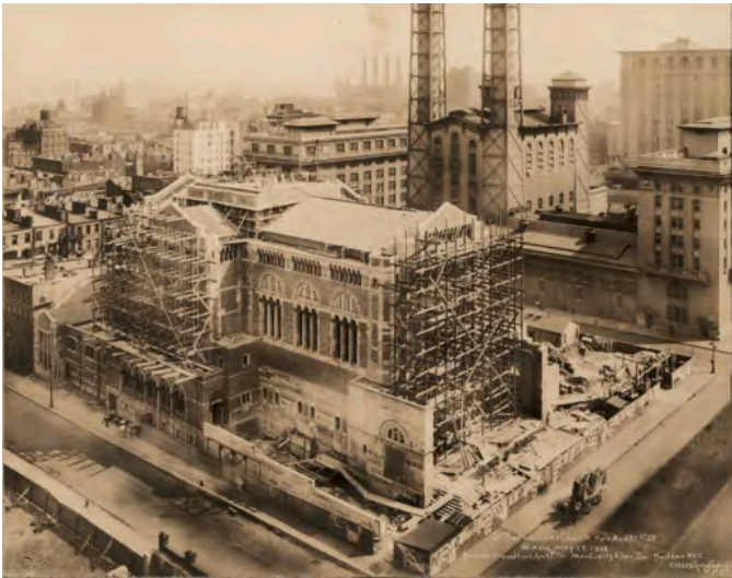
Construction of St. Bartholomew's Church on Park Avenue, 1918
